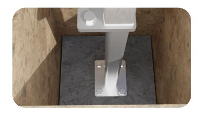
3) Attach the device to the foundation - use 4 M14x100 expansion bolts.
